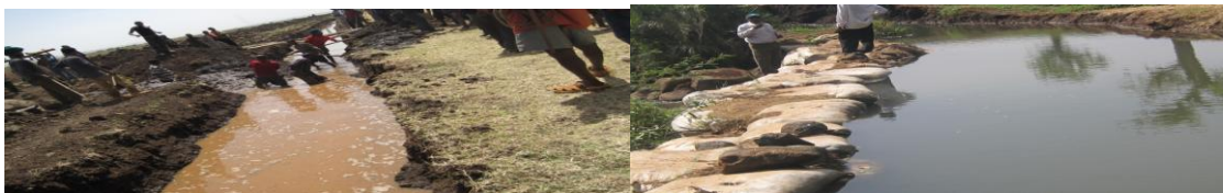
Fig. 6. Labor and material intensive traditional diversion, Fetam River
