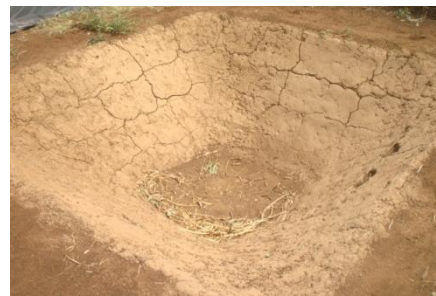
Fig. 8. Shape of cement+soil lined pond
