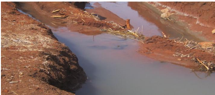
Fig. 8. Uncontrolled water distribution, Silala river diversion, Burie
