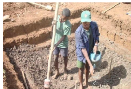
Fig. 6. Clay re-filling technique used
