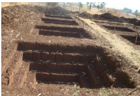
Fig.5. Step by step digging procedure
